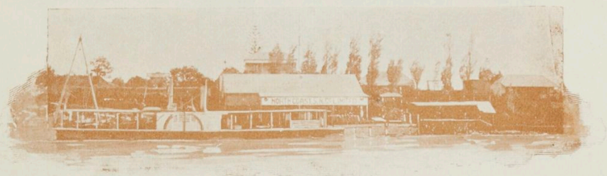
The North Coast Co.'s Wharf at Taree.
