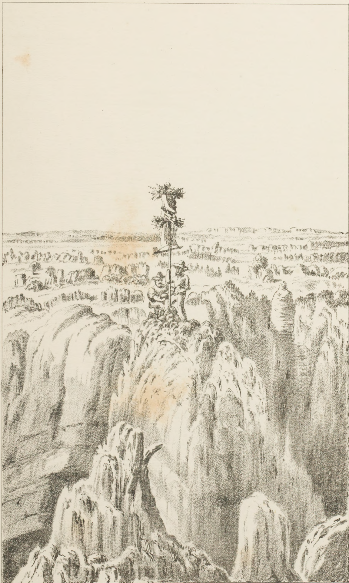
Pl. 15.—Erecting a "Trig." Station on Rough Range.
