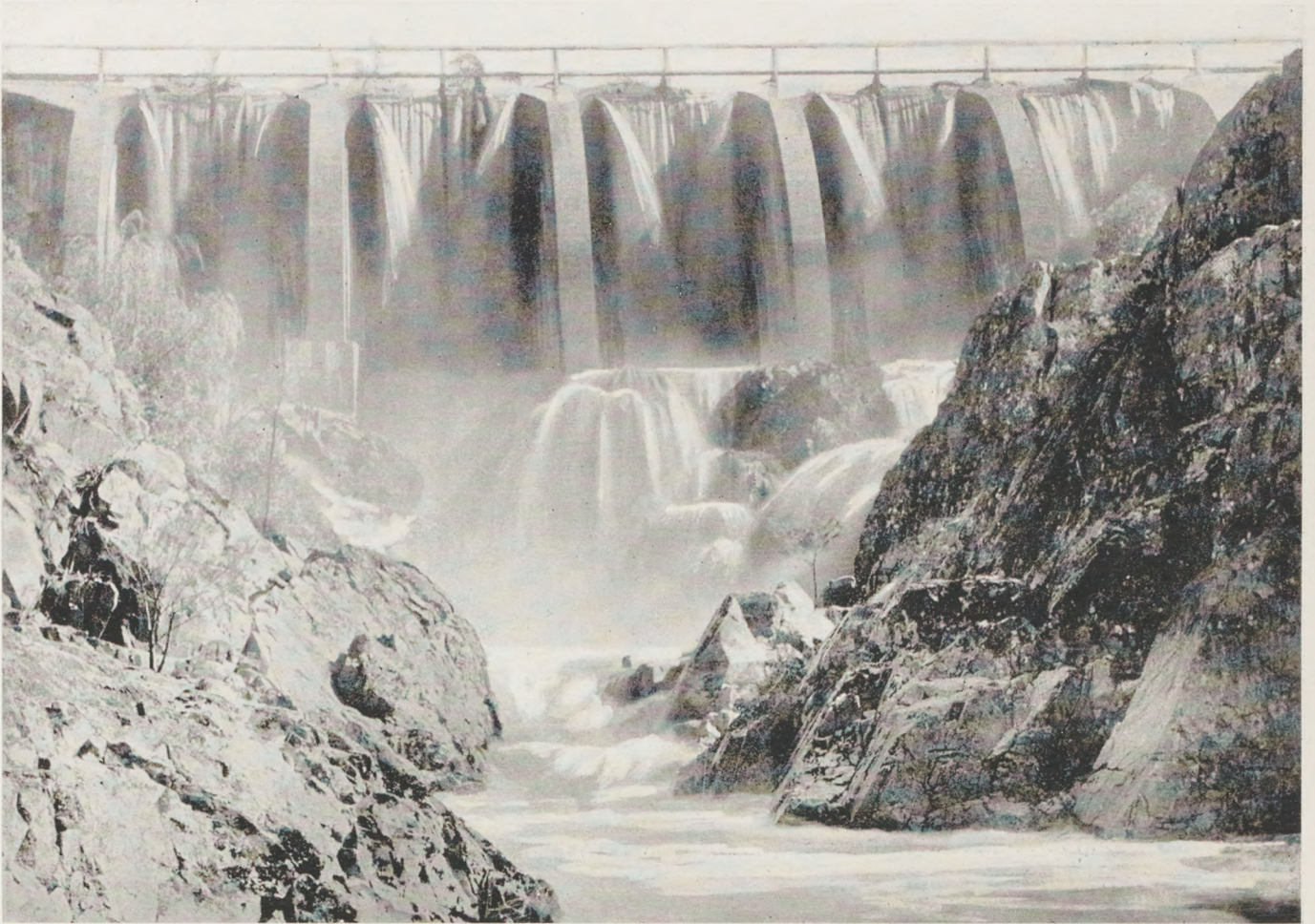
CARCOAR-GARLAND.—“THE JUNCTION DAM” BELUBULA RIVER, SHOWING DRAPERY AND CURTAIN EFFECTS, IN THE PASSAGE OF FLOOD WATERS OVER THE SAME.
