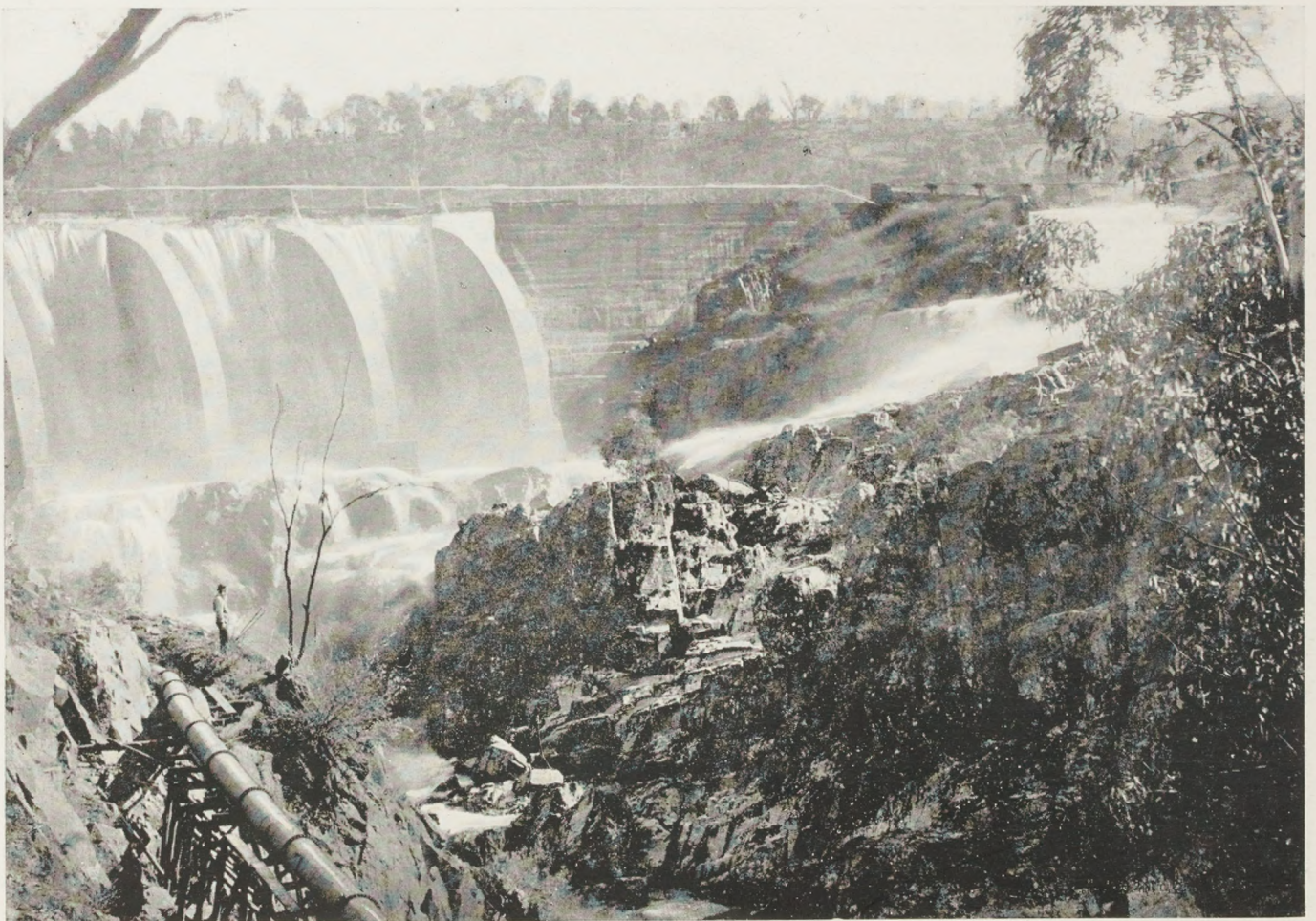
CARCOAR-GARLAND.—“JUNCTION DAM,” BELUBULA RIVER, SHOWING BY-WASH AND PIPE-CONVEYING POWER TO THE 50-HEAD BATTERY AND PLANT OF THE LYNDBURST GOLD-MINING CO.
