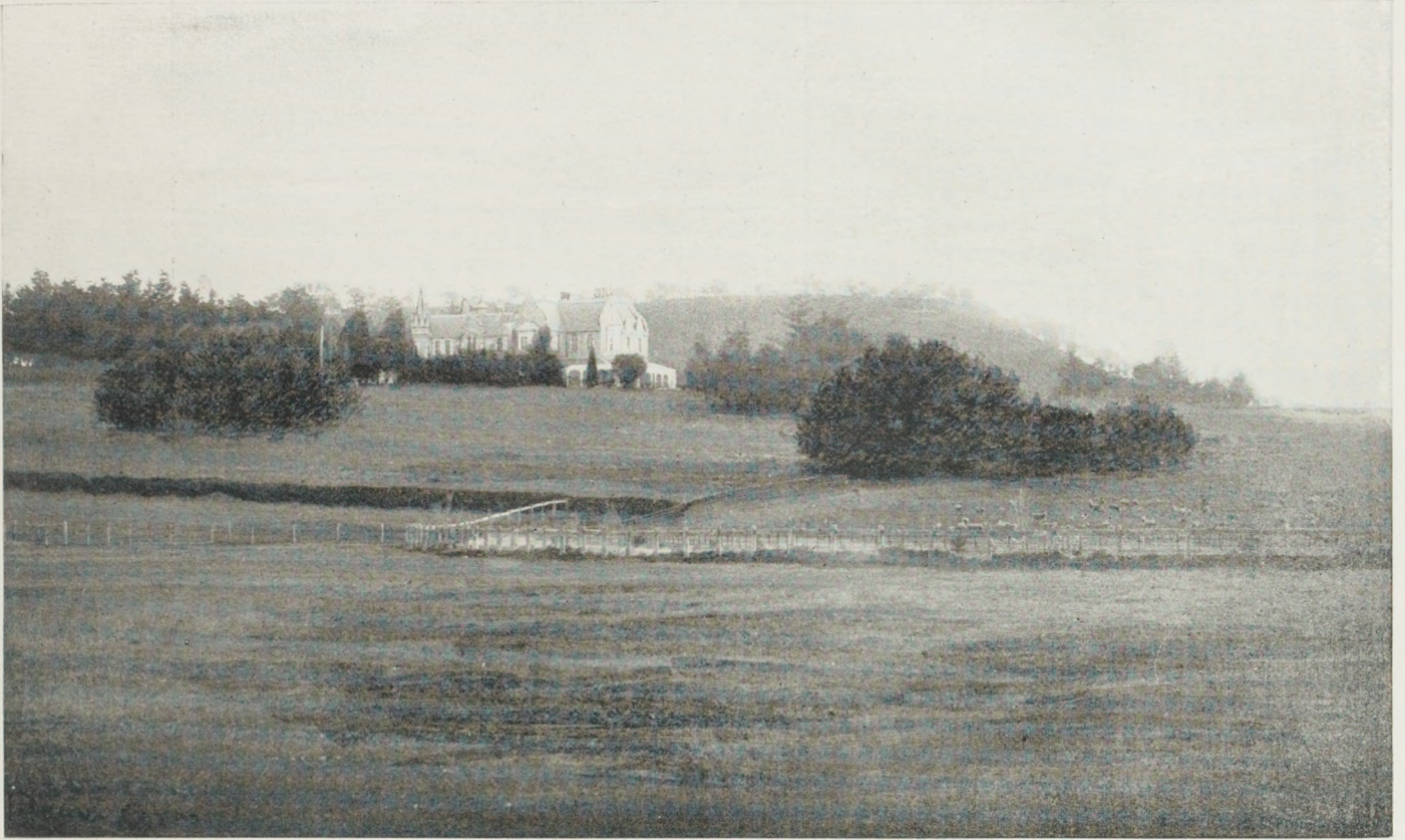
BATHURST.—'THE MOUNT,' RESIDENCE OF J. H. STEWART, ESQ. (STONE USED IN BUILDING OBTAINED ON ESTATE.)
