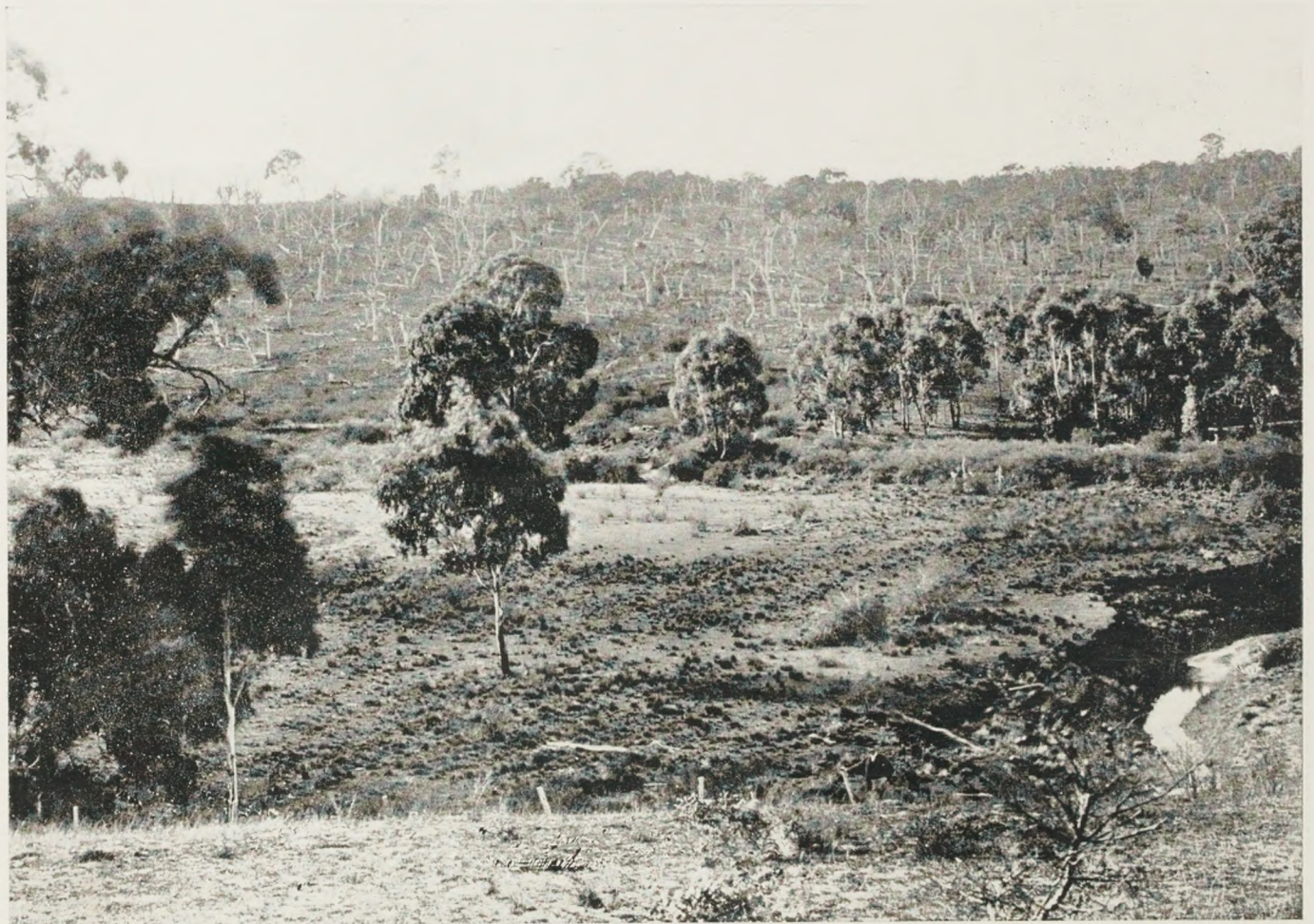
CARCOAR-GARLAND.—PROPOSED RESERVOIR SITE (WATER SUPPLY)—JUNCTION OF MCKENZIE'S FLAT AND BROWN'S CREEK.
