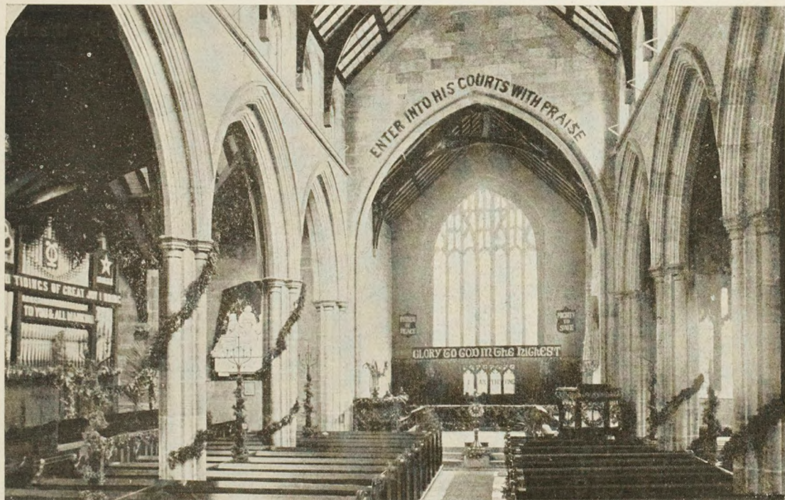
Interior St. Philip's Church before renovation (1885), Christmas.
